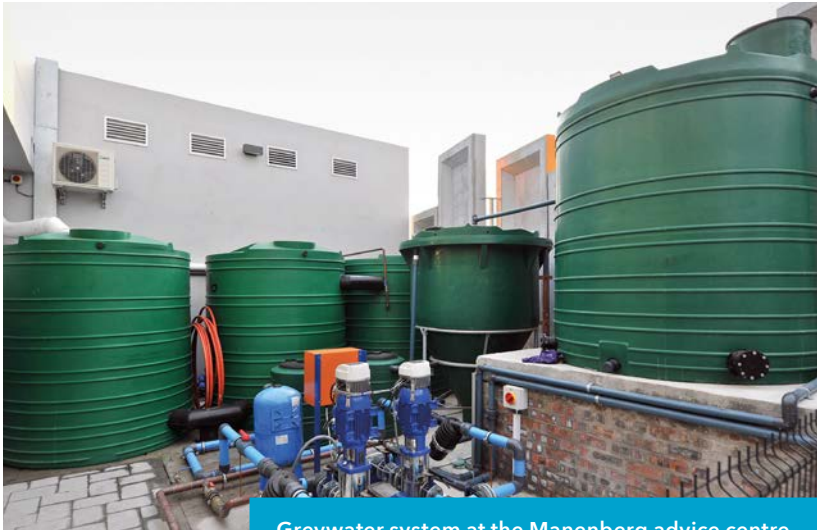
Greywater system at the Manenberg advice centre
