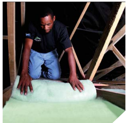
Laying insulation in a ceiling space
